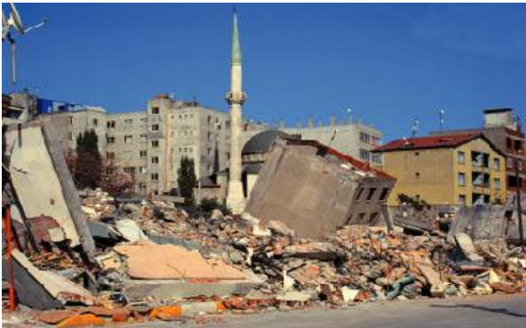
Şekil 1. Deprem rezonans hasar örnekleri(URL-3). Fig. 1. Earthquake damage resonance samples.
